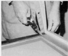
Step 8. Cut off the excess screen with a knife, household shears, or tin snips. A razor blade will also work for plastic. Nail the loose end.
