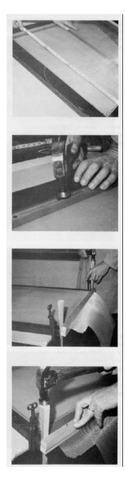
Step 3. Cut the new screen to the width between the shoulders on the frame and 5 to 6" longer than the frame.
