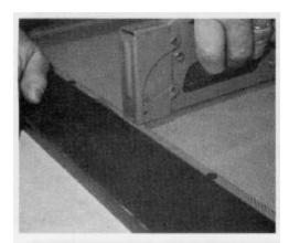
Step 7. Nail or staple the screen fabric on all four sides of each panel about every 4" to 6".
