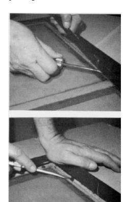
Step 1. Remove wood strips covering the edge of the screen. Be careful not to break them. Pry up with a screwdriver close to the nails to prevent cracking the strip.
