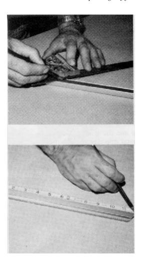
Step 1. Mark off a 45° angle near one end of the material.
